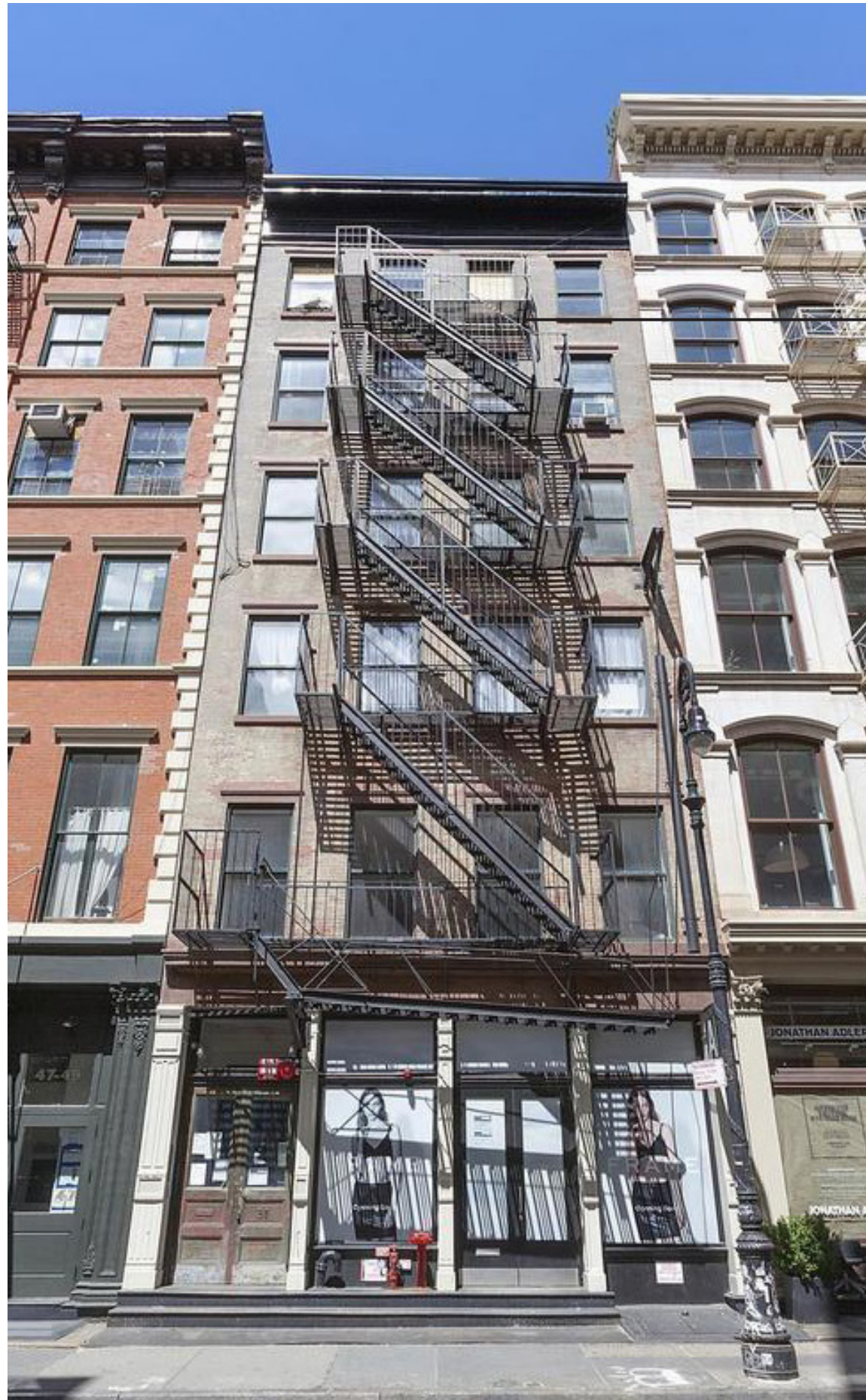
Existing Fire Escape Stops on 6th Fl
