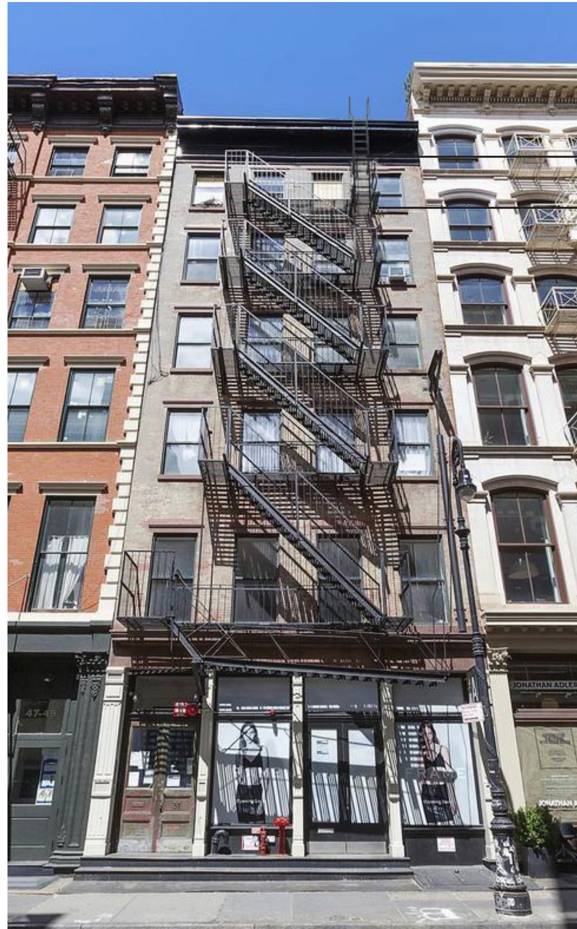
New Ladder to the roof Fire Escape Extension on 6th Fl
